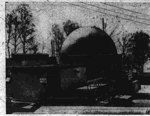
Portable Atomic Plant The Army is showing off its new Atomic power plant which boasts 1,855-kilowatt output and is de signed so components can be shipped by air to remote bases such as the Arctic. The unit is now located at Ft. Belvoir, Va.
